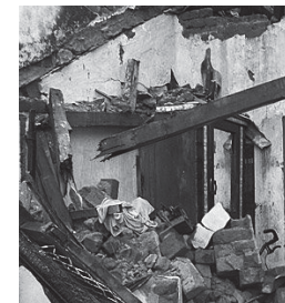
A house damaged by Cyclone Phailin
