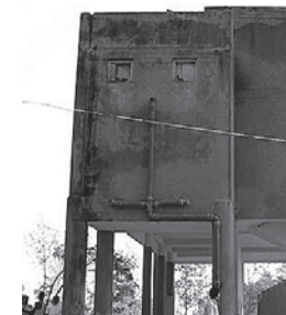
A multipurpose cyclone shelter in Padampur
