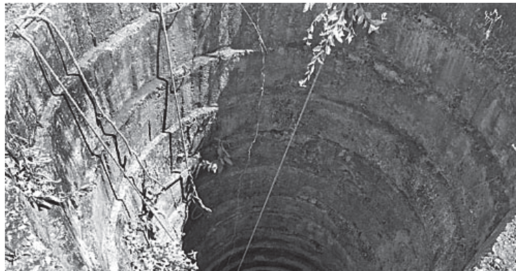
The three bodies were found floating in this well on February 16, at a villager's farm, near National Highway 6 in Bhandara
